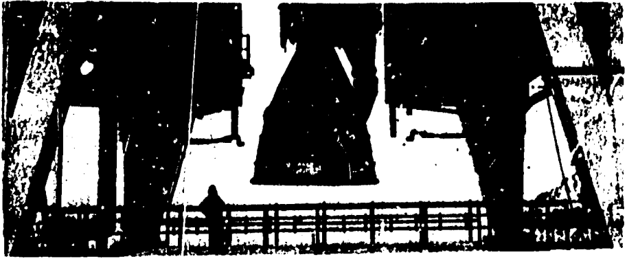
F-1 engine and test stand
