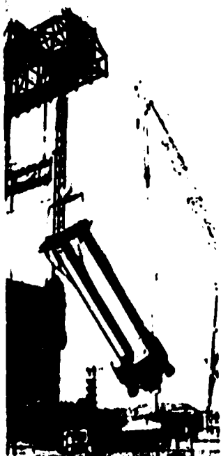
Installation of SA-T2 on static test stand
