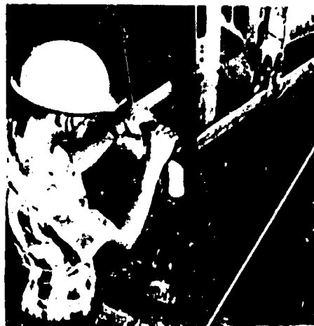
Michoud mechanic drilling holes in the first S-IC lower thrust ring
